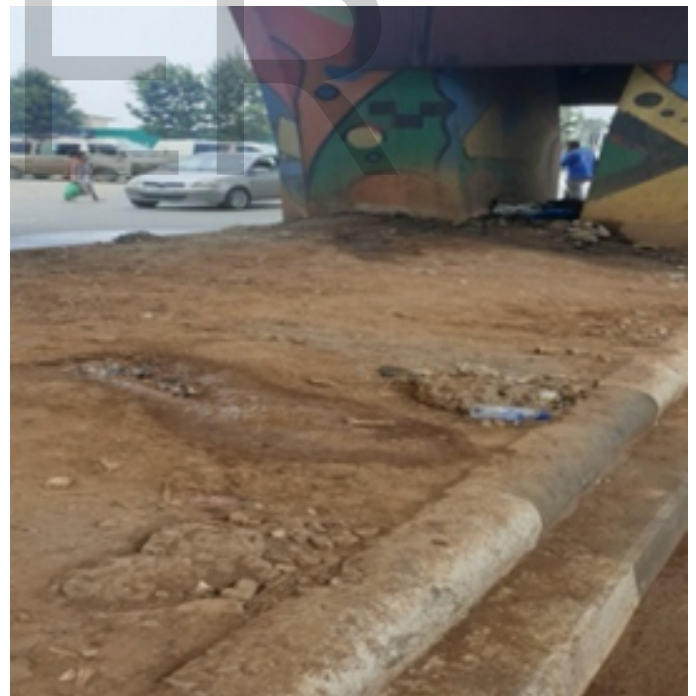
Figure 25: Picture: Under bridge uls
